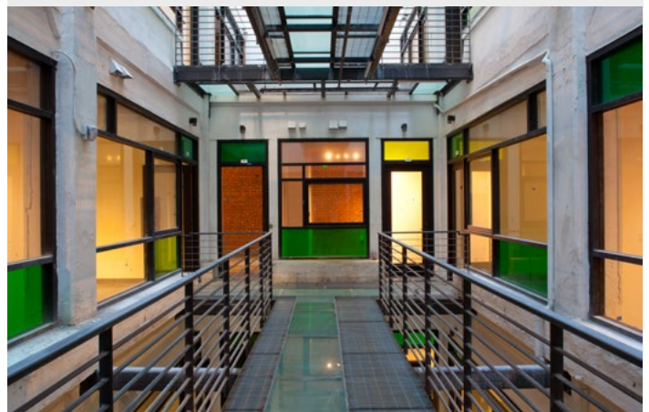
Broadway Lofts (Morgan and Walls, 1906) renovated by Omgivining Architects.
