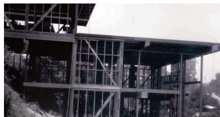
The Wirick House under construction. Photo: Courtesy Barbara Wirick
