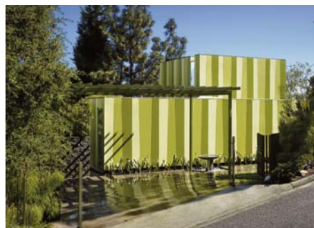
Lago Vista Guest House by Aleks Istanbullu Architects. Photo: David Lena
