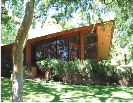
Ablin Residence by Frank Lloyd Wright. Photo: John Berley (4)
