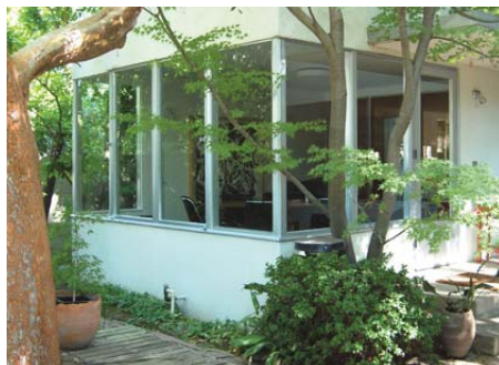
Neutra's Davis Residence (1937).
