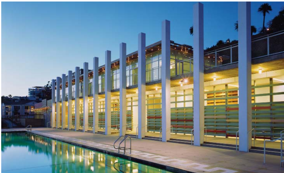
Annenberg Community Beach House (2009) by Frederick Fisher and Partners Architects. Photo: Grant Mudford
