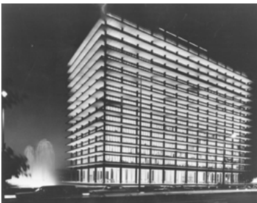
Downtown LA DWP (Albert C. Martin and Associates, 1965).
