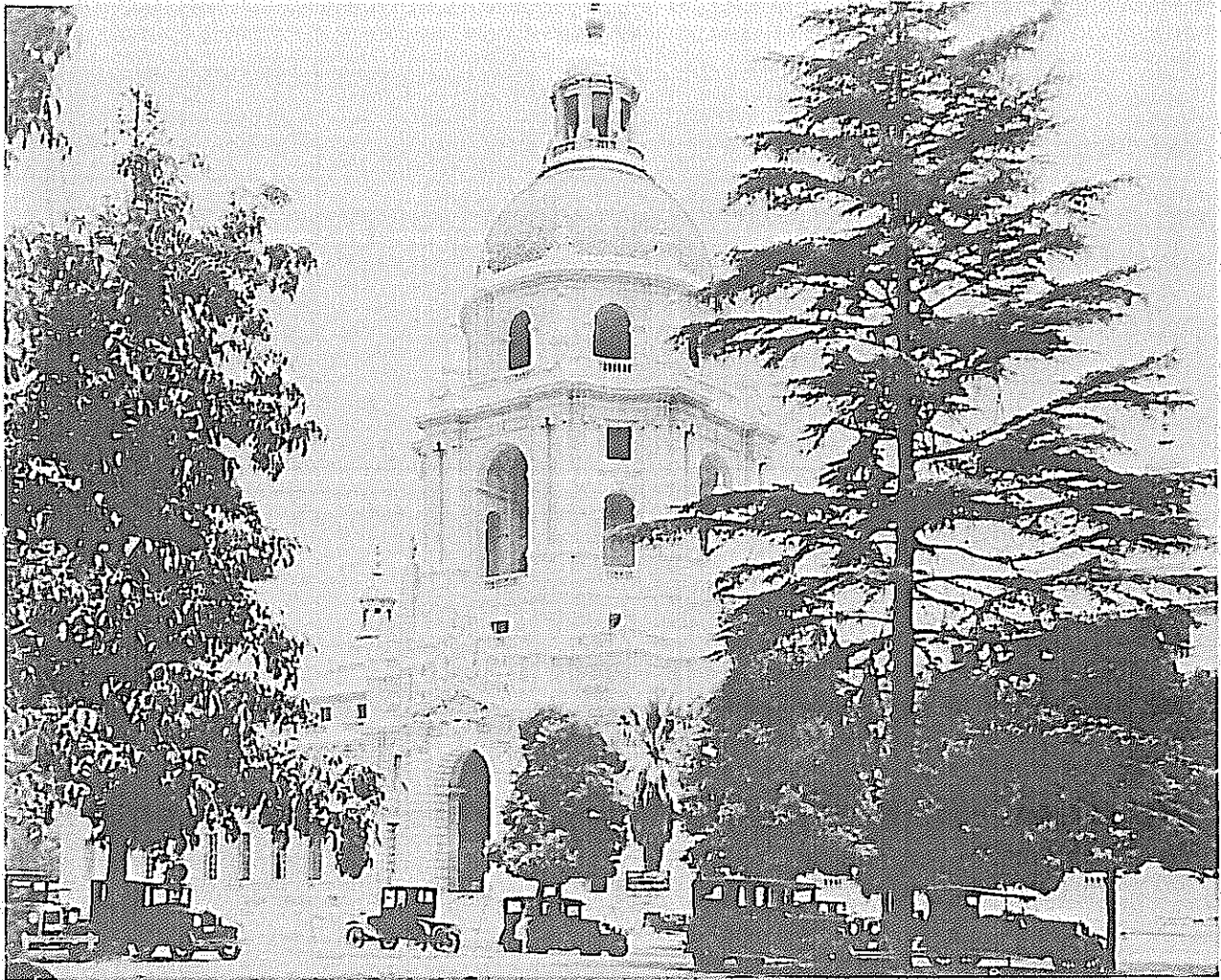
Bakewell and Brown's final design for Pasadena City Hall, with a dome. Source: Urban Conservation Department, City of Pasadena.
